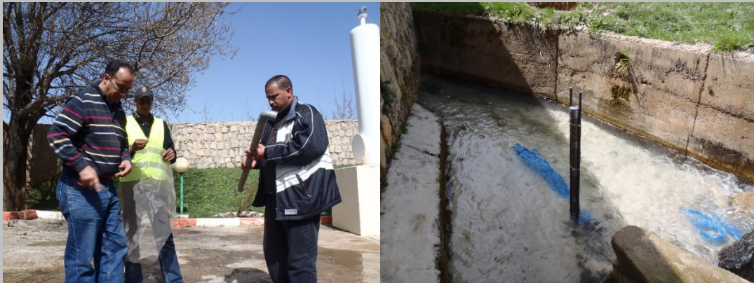
Wrapping a stilling well with filter cloth prior to installation (left); stilling well after installation in spring run (right). Location: Sidi Rached spring near Azrou, Morocco.
