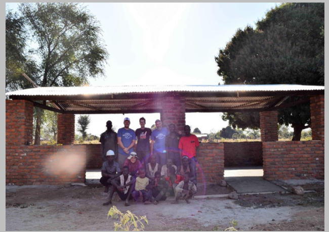
New kitchen facility
